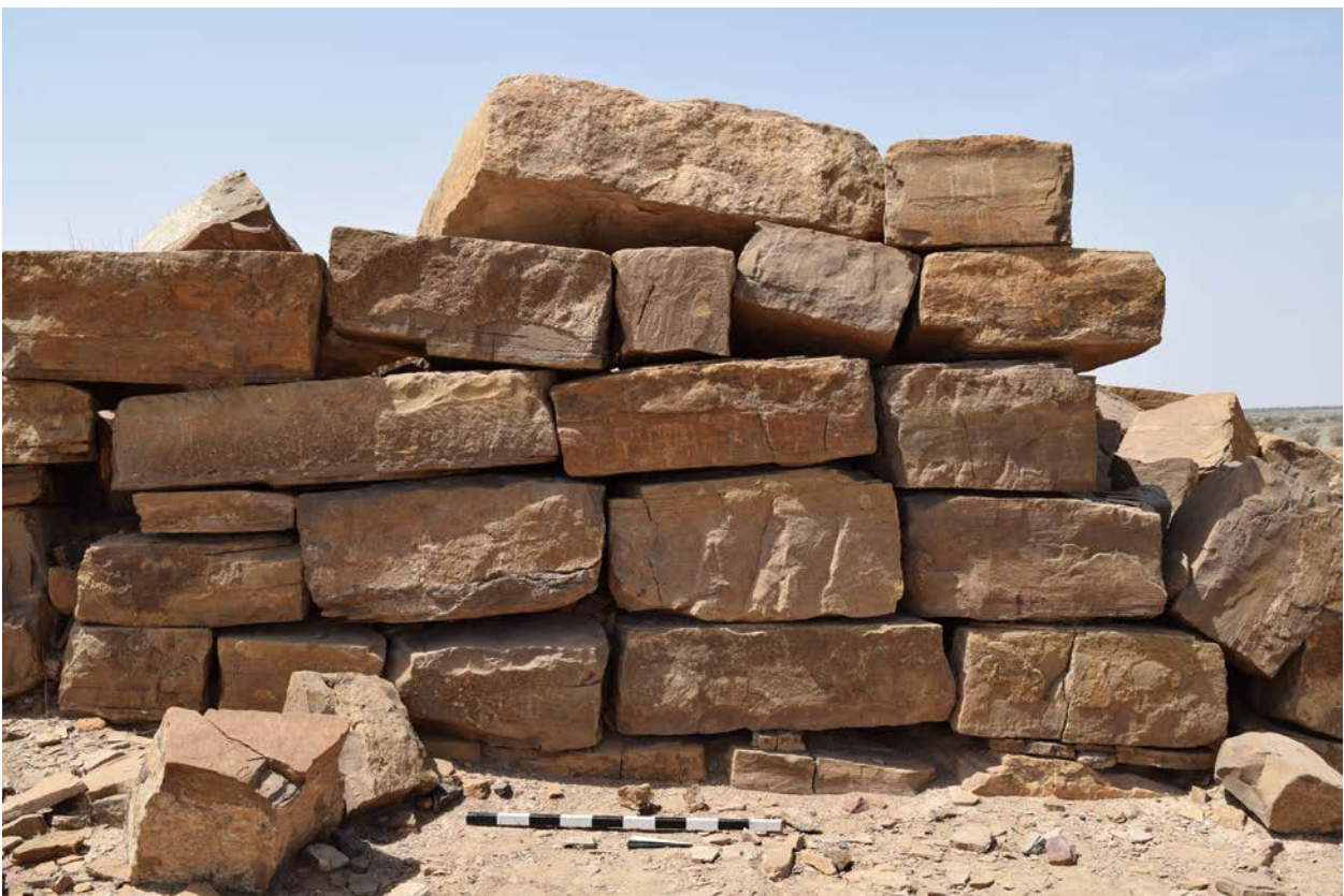
Figure 1.173. Detail of external wall of Building IV.
