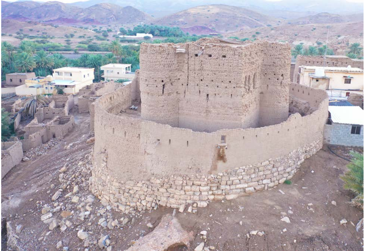
Figure 1.82. A view of Al-Wardi castle and mudbrick ruins in Bat to the southeast. The stone foundation of the tower in the foreground shows a marked change in plan where its original Bronze Age foundation was split open, like segments of an orange, to expand the size of the original structure.
