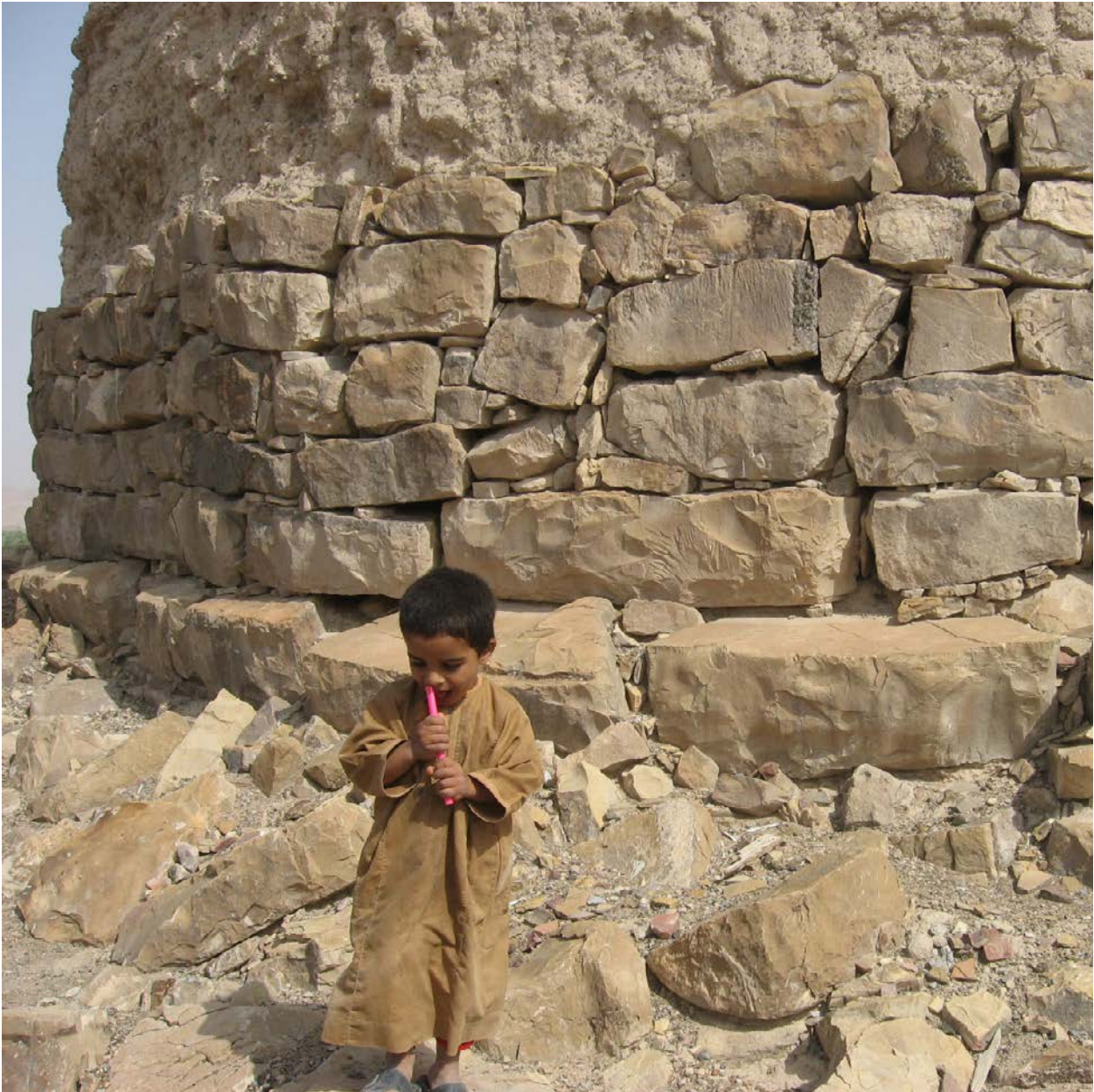
Figure 1.69. Northern “corner” of Al-Wahrah tower showing the large, evenly sized Bronze Age foundation stones beneath the more irregular reconstruction/reuse.
