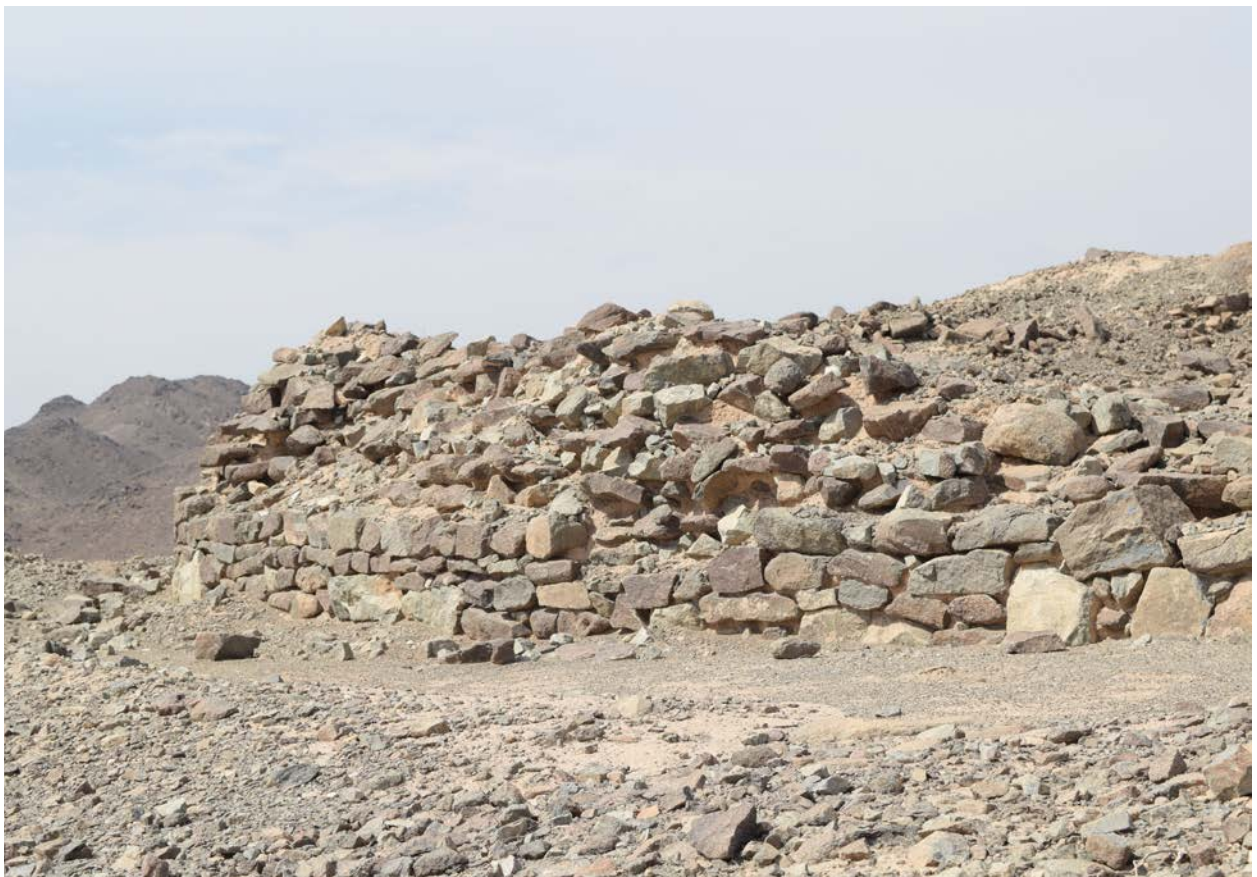
Figure 1.159. Detail of external ringwall of tower Maysar-25.
