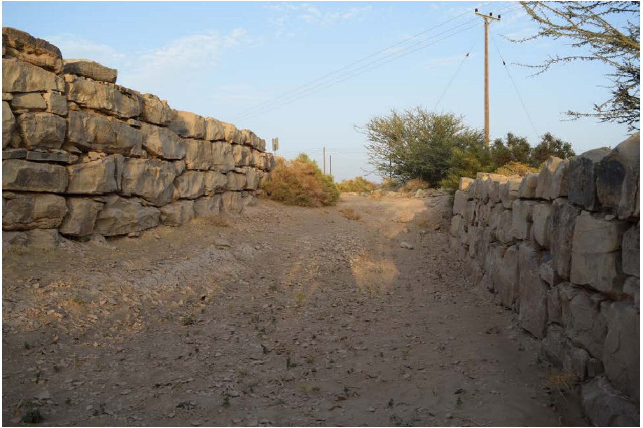
Figure 1.113. Detail of the stone-lined ditch.
