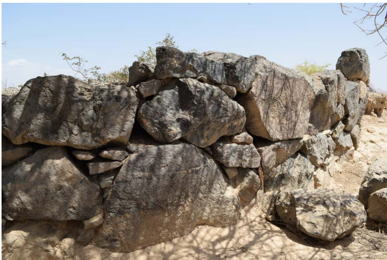
Figure 1.106. Detail of external ringwall.
