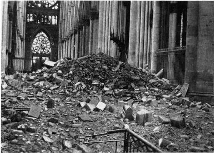
Figure 1. Interior of Reims Cathedral following bombardment in September 1914, which destroyed the framework of the nave and its 15th century lead roof. Single shells continued to strike the ruined building for several years despite repeated pleas by Pope Benedict XV. A major restoration project began in 1919, led by Henri Deneux, Chief Architect of the Service of French Historic Monuments. Image from The Flickr Commons (no known copyright).
