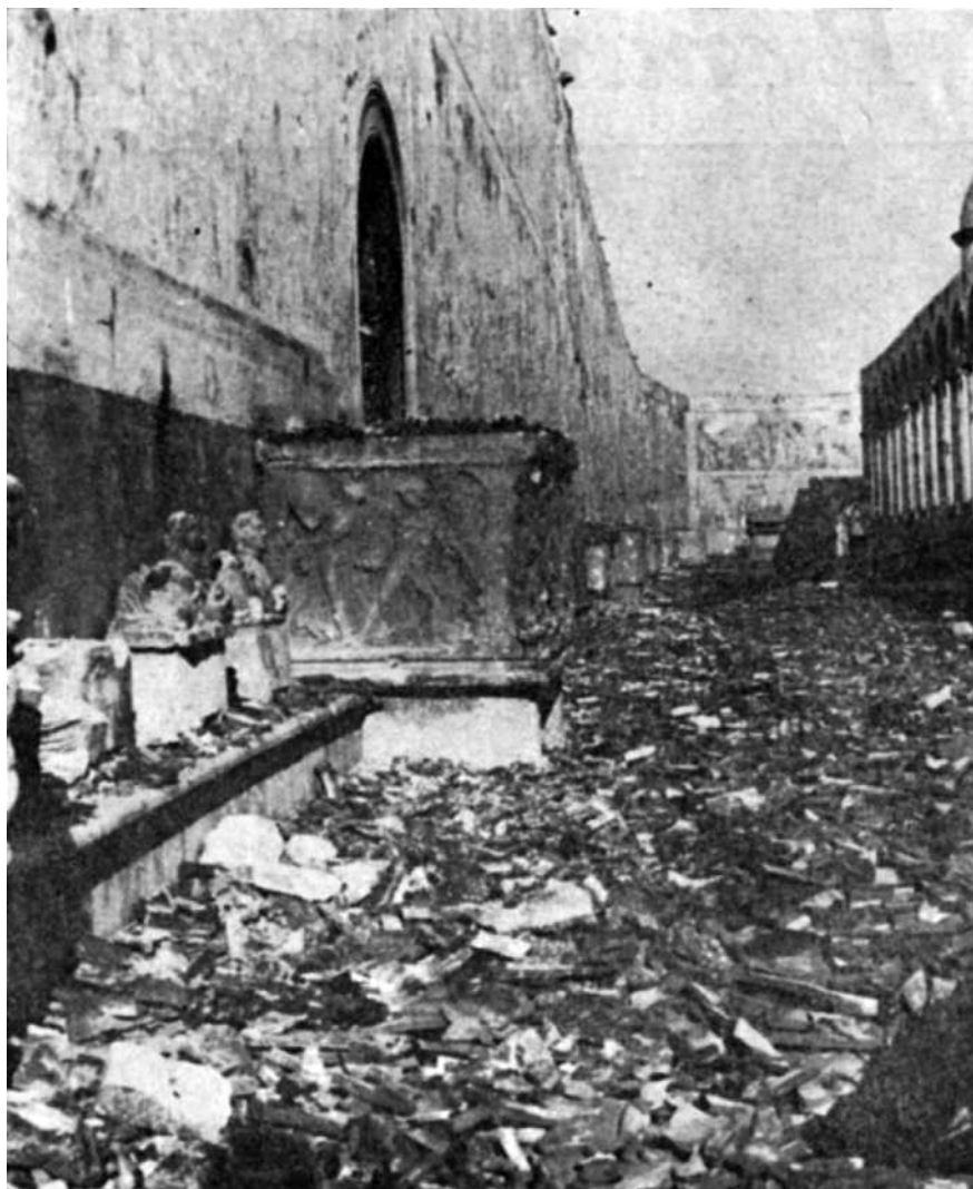
Figure 1. Campo Santo (Pisa) after wartime damage, 1944. Campo Santo's wooden roof was destroyed completely by a fire caused by a bomb that fell in close proximity. Opera della Primaziale di Pisa, via Wikimedia Commons.
