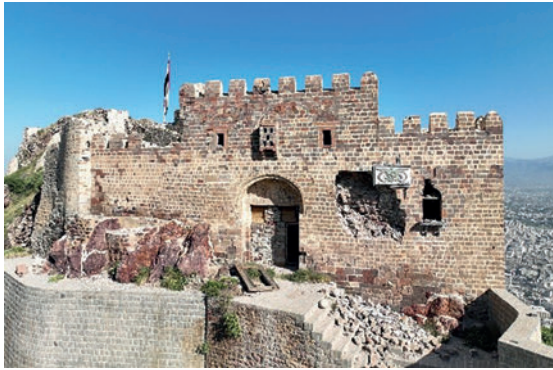
Figure 5. (a) Al Quahira Castle, Yemen, with conflict damage, November 2023. Courtesy of Heritage for Peace (Isber Sabine).
