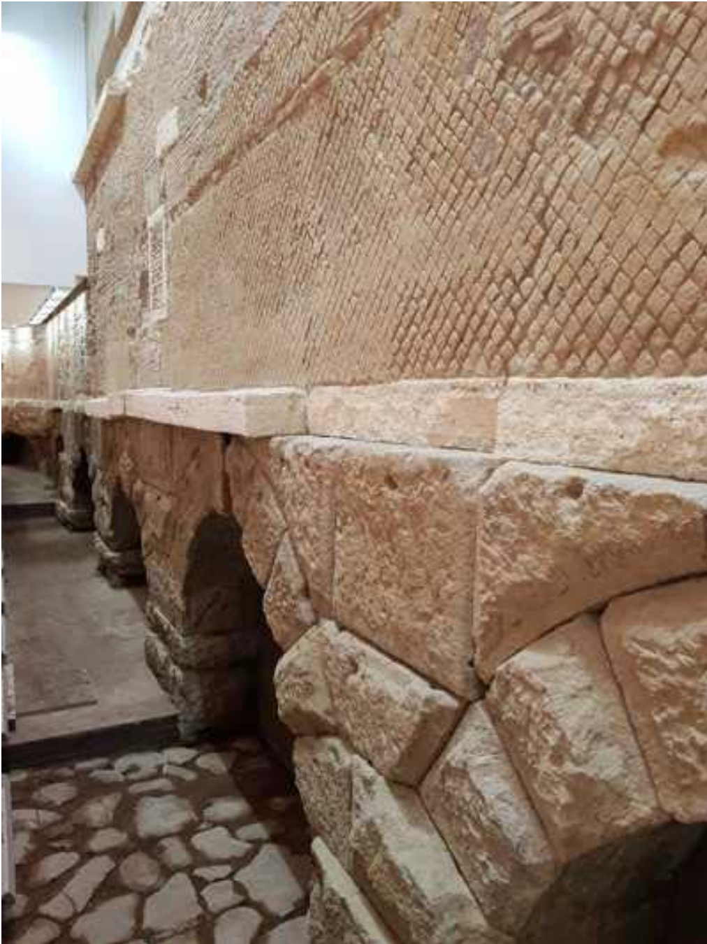
Figure 1. Rome, Aqua Virgo pipeline, I c. b.C., refurbished during the Middle Ages. ©2023 Francesco Salvestrini.
