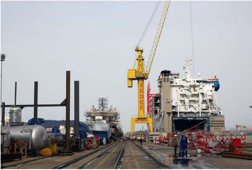
FIGURE 1.4. Sedef Shipyard, Tuzla, Istanbul, 2018. The bright-yellow crane used in the building process reads “Sedef: Önce Emniyet,” meaning “Sedef: Safety First” in Turkish. Photo by the author.
