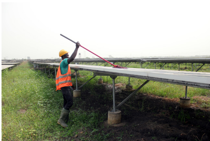
FIGURE 3.1. Man with a mop cleans dust and mud from solar panels during harmattan, Meinergy solar power station, Winneba, Ghana, 2020. Photo by the author.
