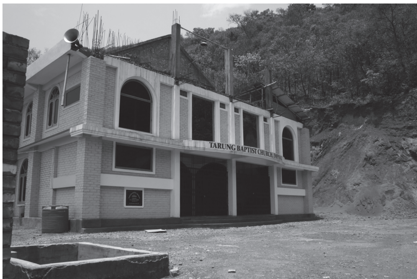
Image 6.2 Baptist church under construction, Langol
