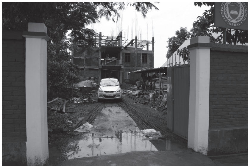
Image 7.1 School under construction, Sangaiprou
