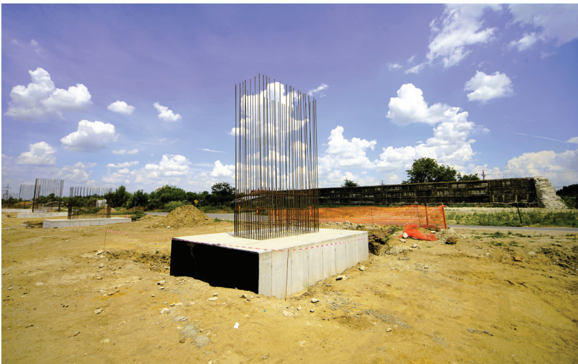
Figure 7.2 In the foreground, the building of a new bridge over the Argeș River as part of a highway project to Bucharest, near Grădiște; in the background, the half-demolished bridgehead of an unfinished socialist bridge over the now abandoned Bucharest-Danube Canal, industrial ruins of a bygone era. Photo: Constantin Iordachi.
