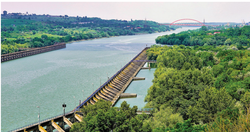
Figure 7.5 The Danube–Black Sea Canal with the Cernavodă Bridge in the distance (built in 2002). Drone Photo: Constantin Iordachi.
