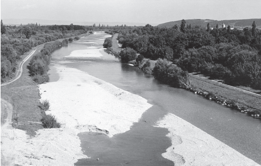
Figure 10.5 The riverbed of the Traisen after the completion of channelization in 1913. The groundsills are visible in the upper section of the picture as well as the large sediment bars, which are above water level due to the residual flow. (© Traisen Wasserverband)
