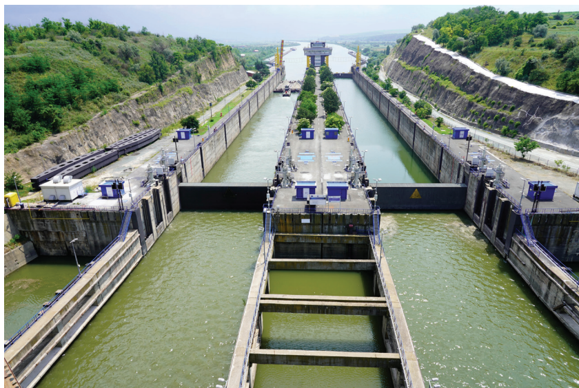
Figure 7.6 Infrastructure on the canal: The Cernavodă Lock, the entry point to the canal (left). Photo: Constantin Iordachi.
