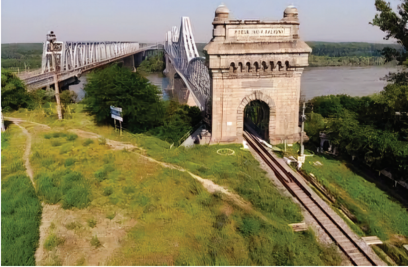
Figure 7.1 The Carol I Railway Bridge over the Danube, which linked Dobrudja with the Old Kingdom (1895) (right); and the Cernavodă socialist railway and freeway bridge (1987), which further amplified but also appropriated, in a socialist key, Romania's modernization project at the Lower Danube (left). Drone photo: Constantin Iordachi
