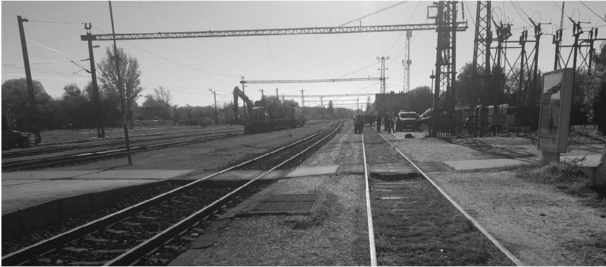
Figure 5.2 Workers remove ageing rail equipment from the extant track outside Budapest
