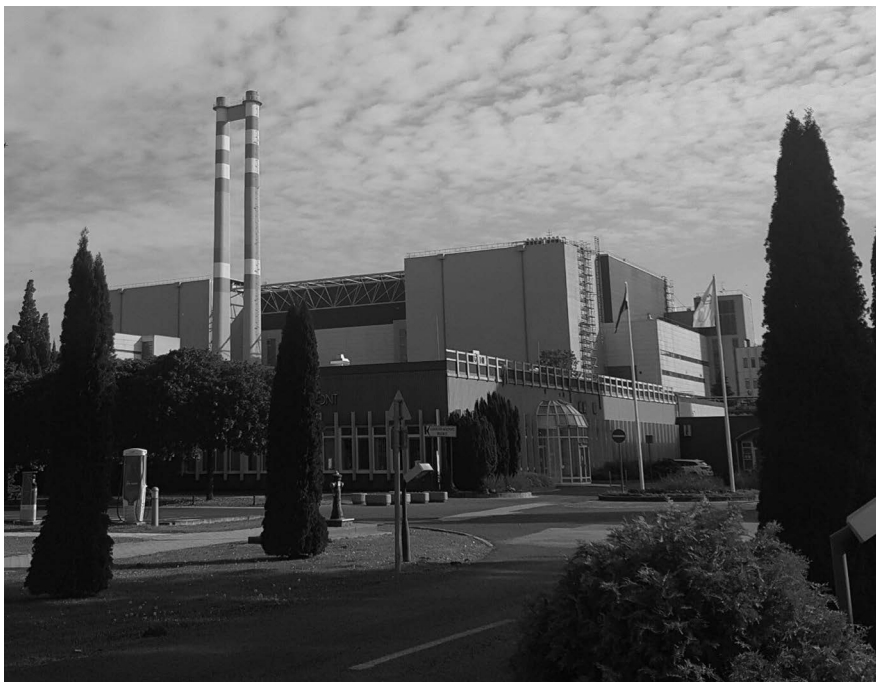
Figure 4.1 The exterior of the Paks nuclear power plant in central Hungary
