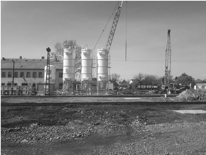
Figure 5.3 The Belgrade-Budapest railway line under development at Soroksár station, southern Budapest
