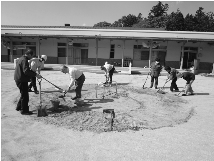
Figure 3.4 Professor Anzai and other volunteers removing contaminated surface soil at Sakura kindergarten, Fukushima City about 60 kilometres from the nuclear power plant, May 8, 2011. Contamination levels were found to be around 100 times higher than normal. Special exhibit Radioactivity and the Future of Humanity , Kyoto Museum for World Peace. Credit: Anzai Science and Peace Office, Fukushima Project for a Safer Future.
